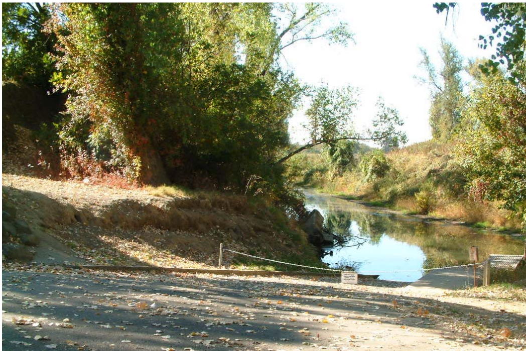
Butte City Launch Facility – currently closed due to channel siltation.
