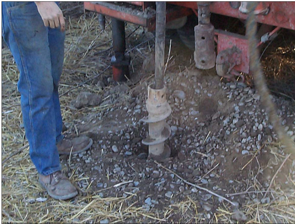
SPT Sampling Through Hollow Stem Auger
